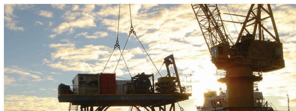
Lifting & Hoisting, including SME documents
