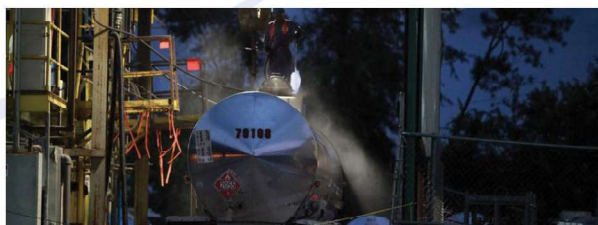
Gas free & Tank Cleaning works
