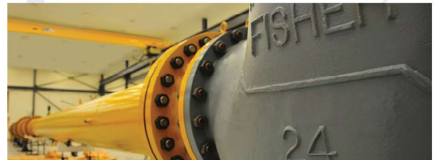
Pressure Testing (Pipelines & Loading hoses)
